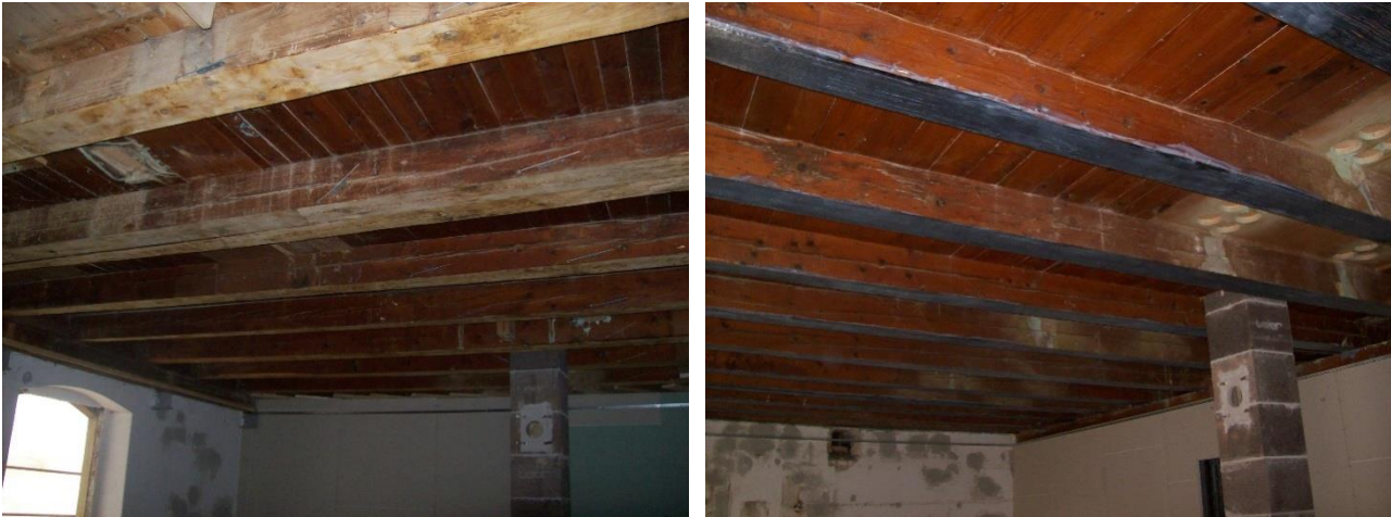
Figure 6 Old timber beams before and after reinforcement
