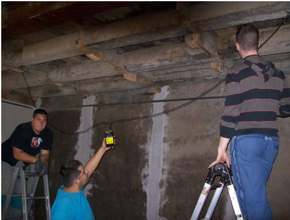
Figure 4 Non-destructive method FAKOPP
