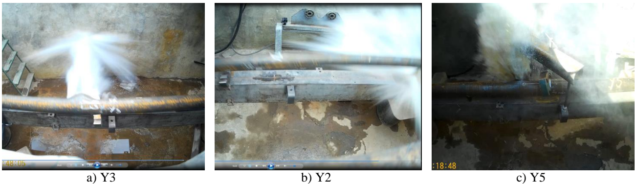
Figure 3 The investigated pipeline sections at the moment of their failures
